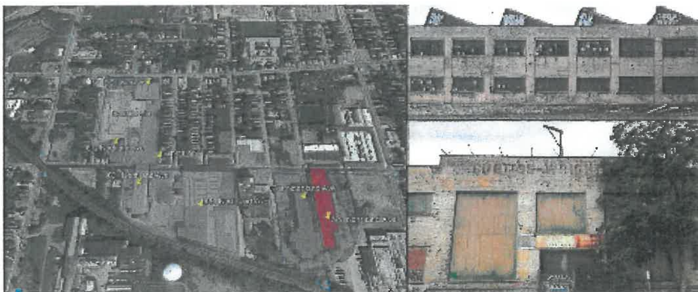
Figure 1.11. 777 Northland. Note: (Clockwise left to right) 777 Northland appears in red on satellite imagery; exterior of saw-tooth roof facing west; historic wall on Northland Avenue to be saved for future building. Source: Google Maps (2020); Justyn Bellitto (2020).
