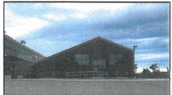
Figure 1.5. The "Red Shed" at Northland Central. Note: Rehab space now occupied by Garwood Medical Devices. Source: Justyn Bellitto (2020).
